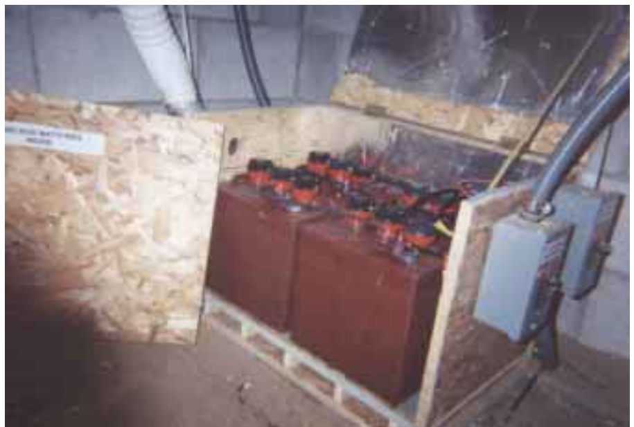
Four Trojan T-105 batteries, 440 AH at 12 VDC. Note the Hydrocaps, DC disconnects, and removable front wall on the box.
