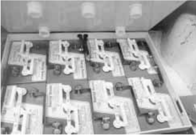
The tubes on the lid of this box press down to hold the batteries firmly in place.
