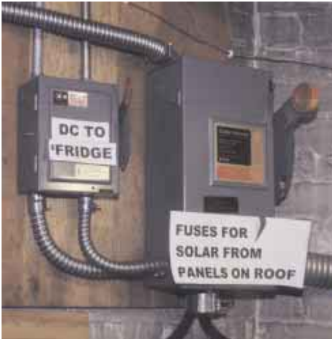
Left: DC distribution. Right: PV disconnect.
