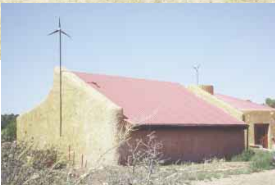
The shop contains the renewable energy system.
