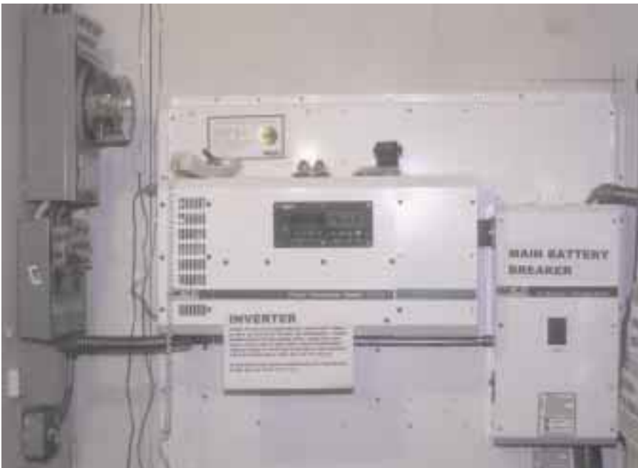
KWH meter shows solar energy produced (left); Trace 2512 inverter.
