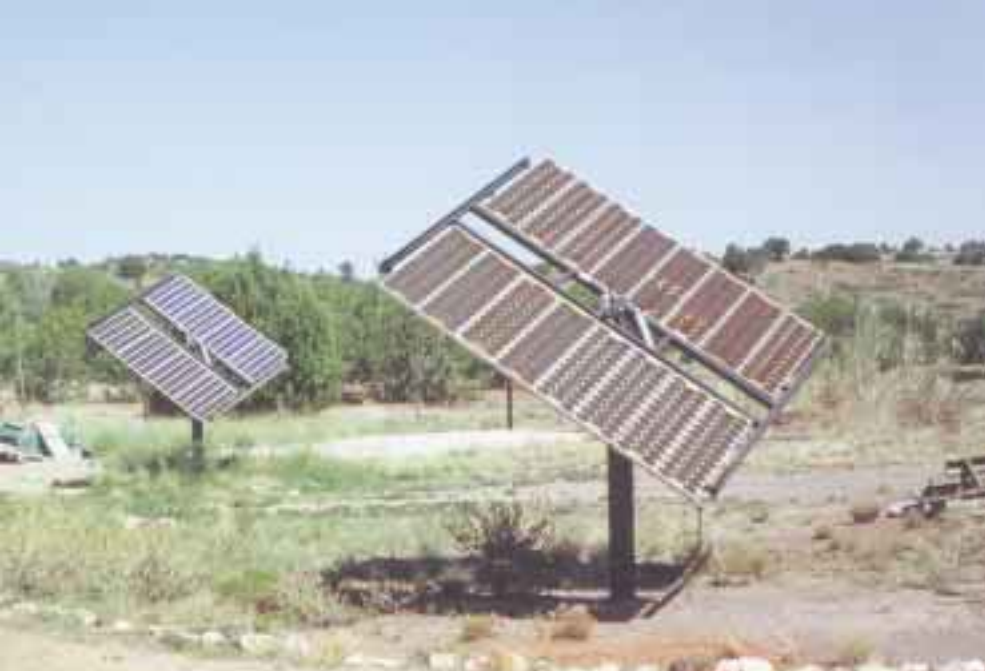
Eight Siemens SP75s and sixteen Arco M-51s on Zomeworks trackers on the north side of the house.
