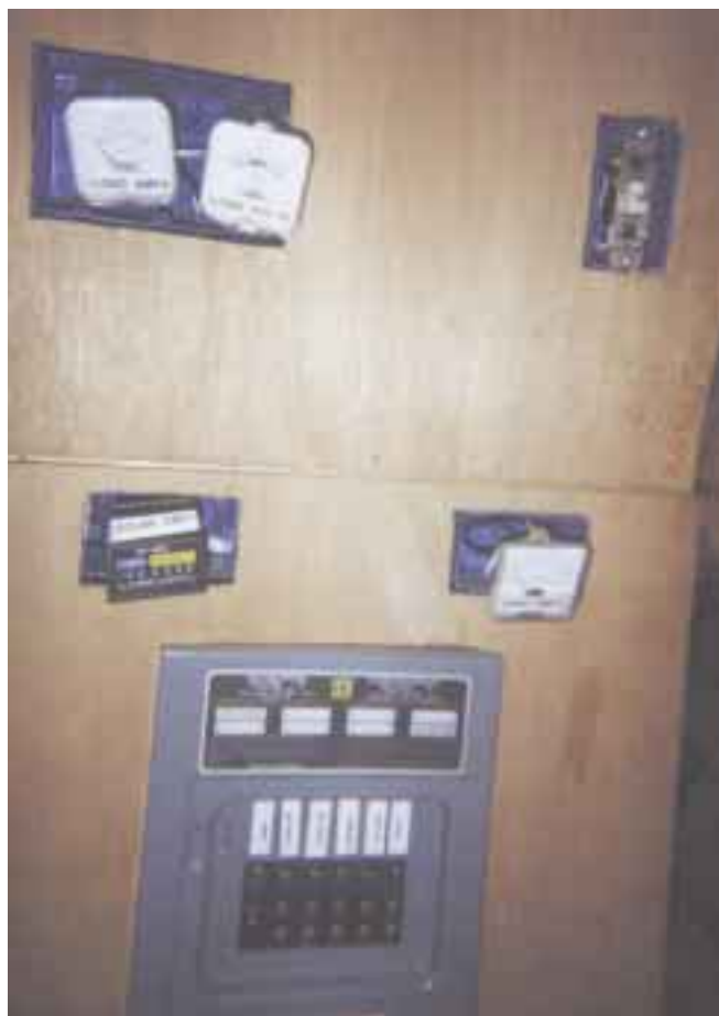
Square D breaker panel with six circuits, DC meters, and wall switch for the 12 VDC light above. Box covers are removed for final inspection.
