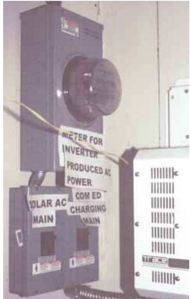
All solar energy is counted with a KWH meter.
