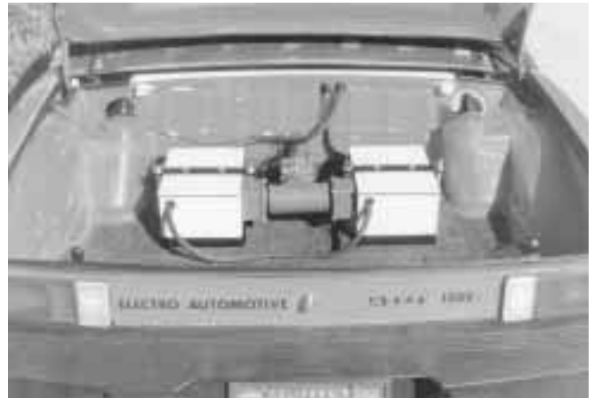
Grey PVC pipe provides fittings for forced air ventilation of boxes during charging.
