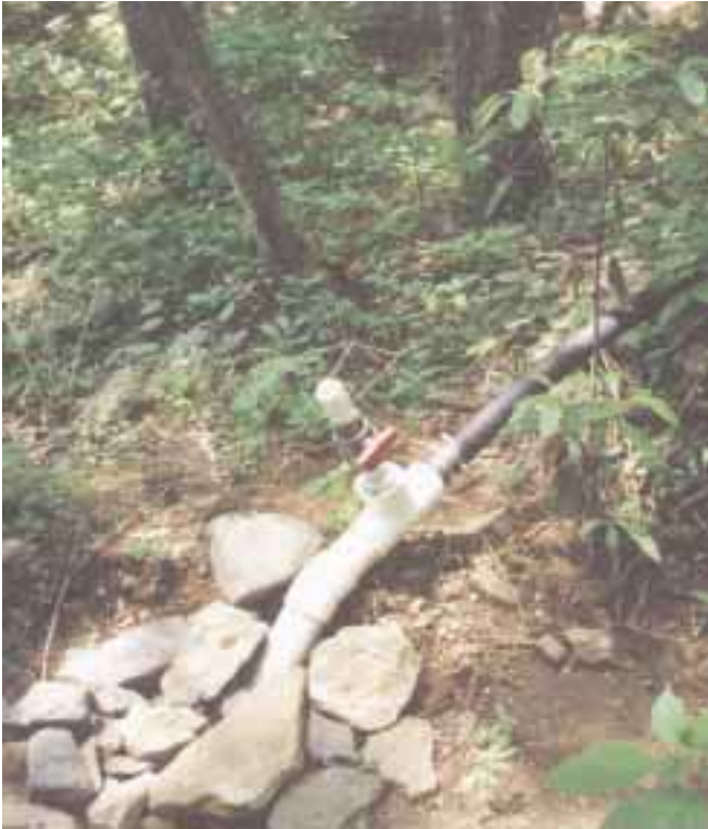
The air release valve between the 600 feet of 3 inch pipe and 400 feet of 4 inch pipe.
